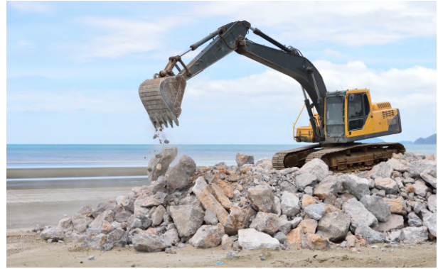
Fig. 1. Fragmented rocks excavation using an excavator.
